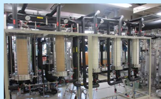
Photograph of fully automated pilot plant for 50 L/day installed last month (Now test operations are being performed.)
