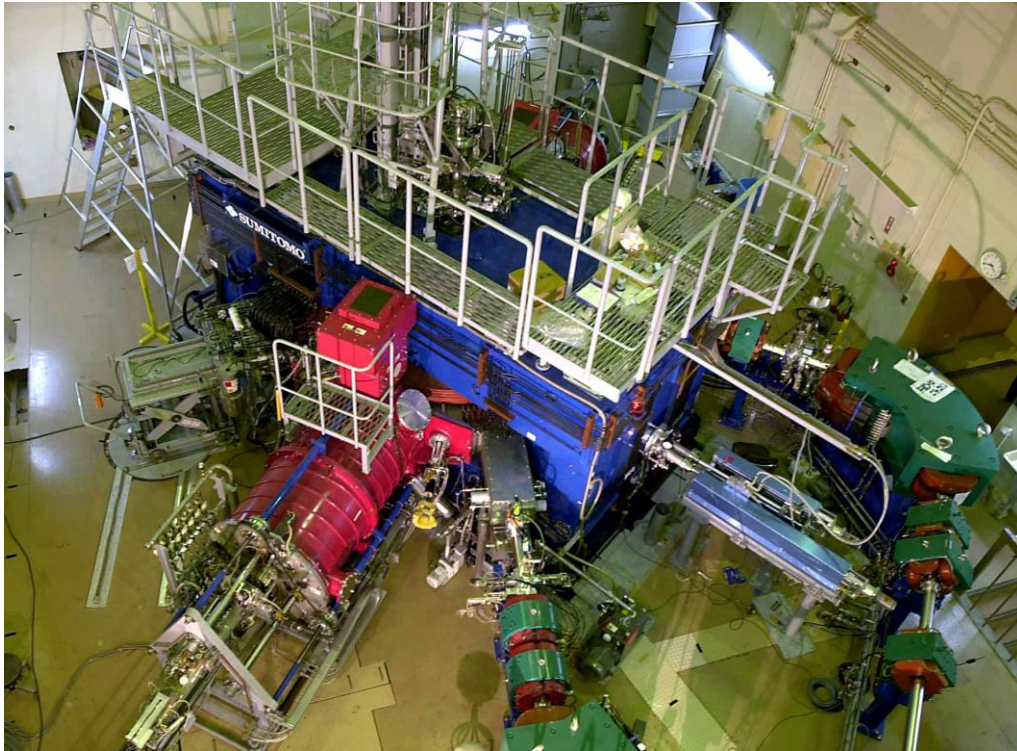
930 AVF cyclotron (Multiple use, K=110)
